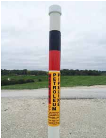
Our pipeline markers can be typically identified by the black and red bands at the top.
